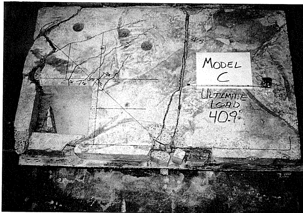
B.) Photograph of Cracking Pattern
